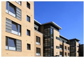
Construction techniques vary across the scheme with a range of differing but complementary materials, featuring traditional brickwork, terracotta rain screen cladding and zinc standing seam cladding and roofing.
