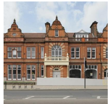
Tottenham High Road, N17
