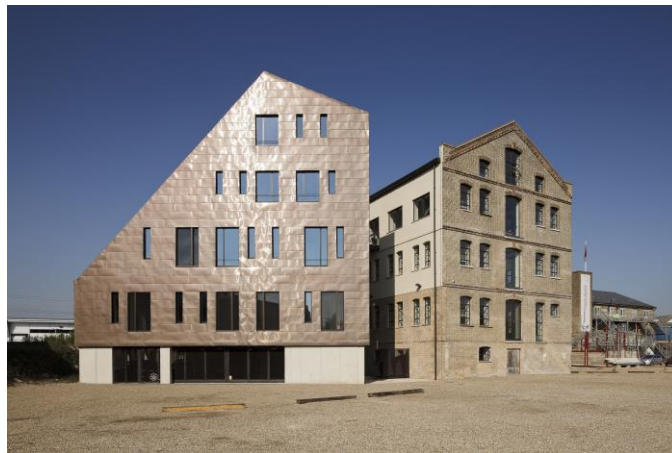
(Rooff head office, The Granary, 80 Abbey Road)
