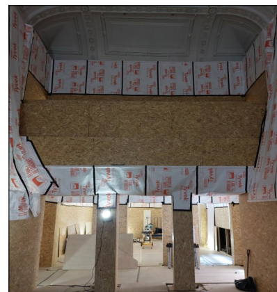
Exposed roof trusses & protection to the Great Hall
