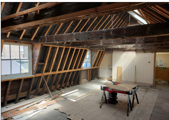
Exposed roof trusses & protection to the Great Hall
