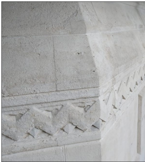
Stone work cleaning
